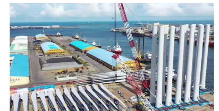
Pre-assembly work conducted at the Port of Taichung in the Changhua Offshore Wind Farm Project
