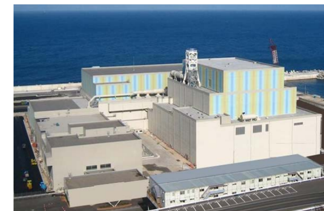
The Chugoku Electric Power Co., Inc., Shimane Nuclear Power Station Unit 3 (under construction)
