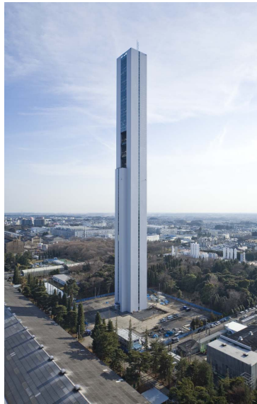
External view of the new elevator research tower
