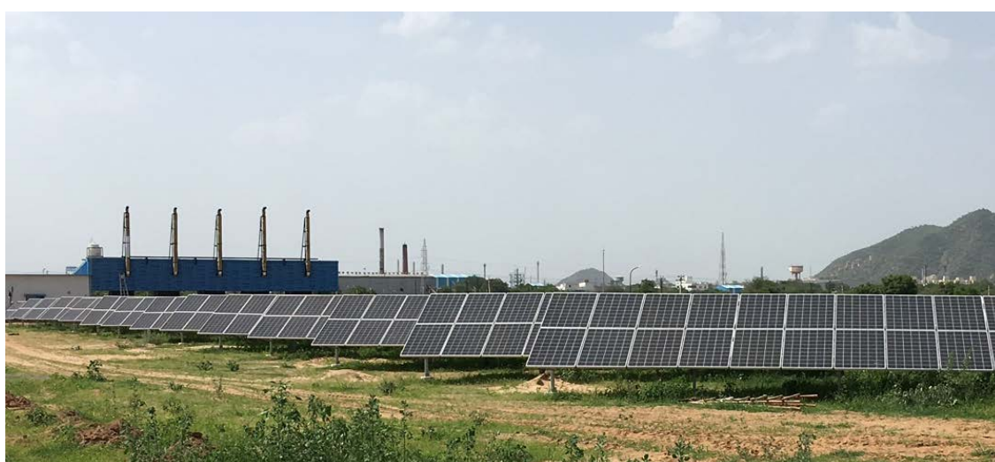
Figure 1. Microgrid system using PV power generation
