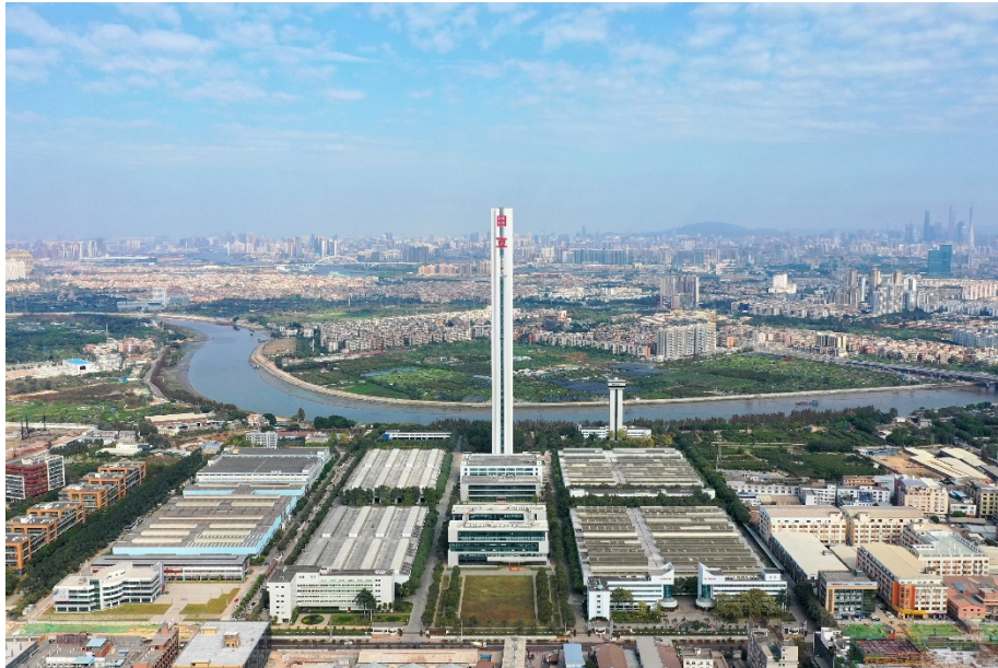
External View of the H1 TOWER
