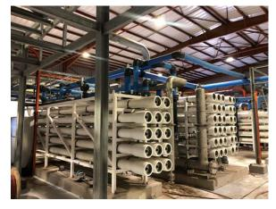
The seawater desalination and water reuse integrated system (Reverse Osmosis (RO) membrane)
