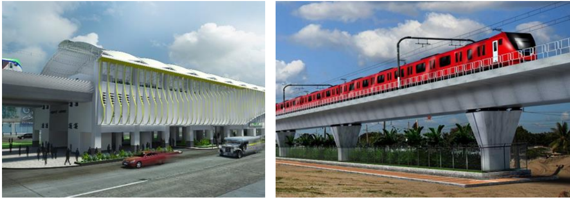
External View of North-South Commuter Railway (Image)
