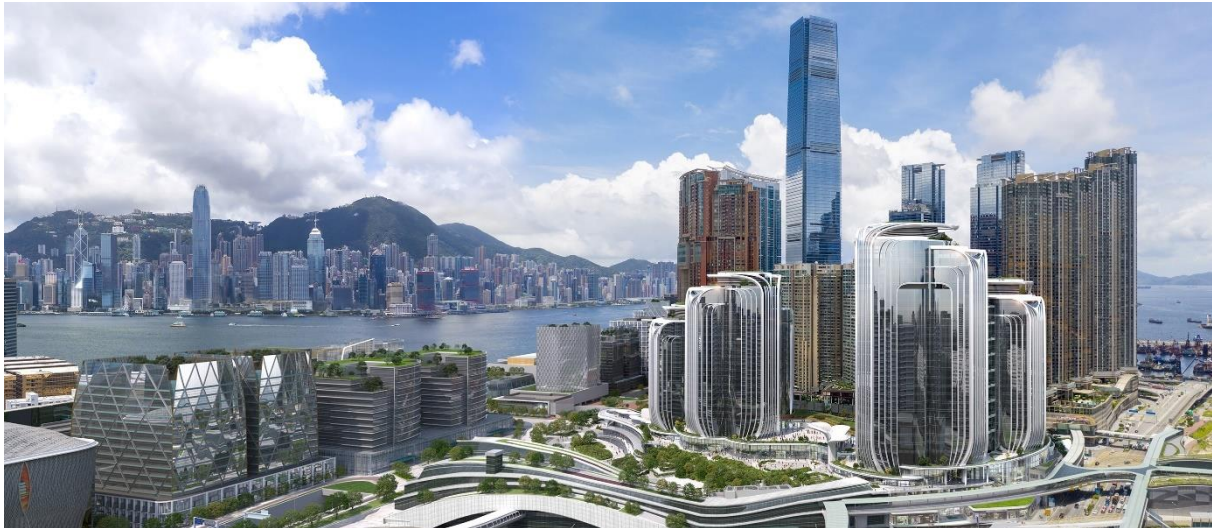
External view of the West Kowloon Station complex in Hong Kong (in the right foreground of the photograph)
