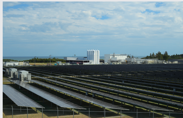
Figure 1 | Fukushima Hydrogen Energy Research Field
