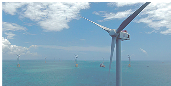
1 Taiwan offshore 5.2-MW wind turbine generators
