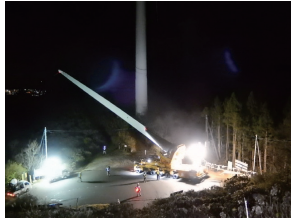
4 Operation of blade lifter
