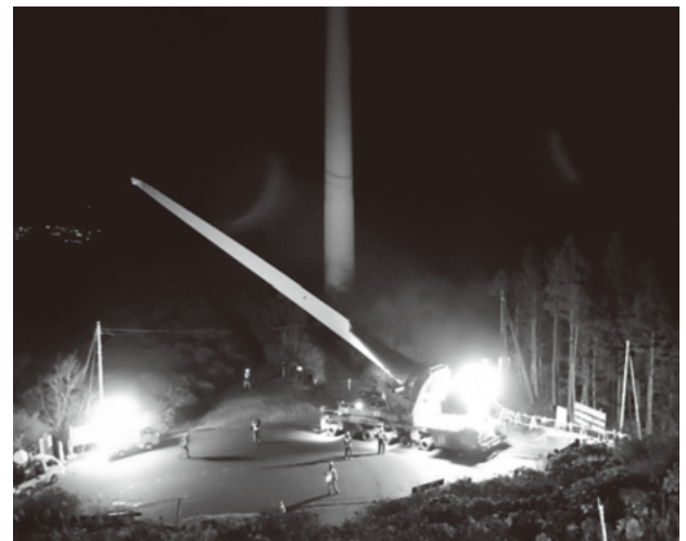
Figure 3 — Blade Lifter in Action Transporting Blade
