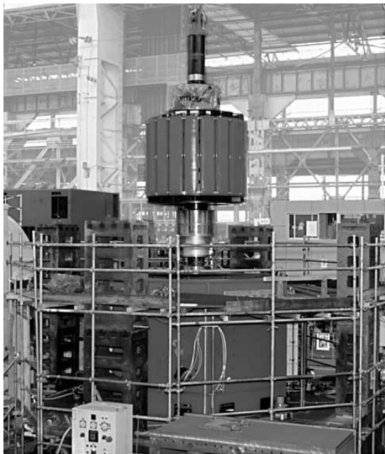
Fig. 5—Plant Assembly of Synchronous Motor. Hoisting of synchronous motor rotor.
