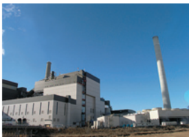
Walter Scott, Jr. Energy Center Unit 4
