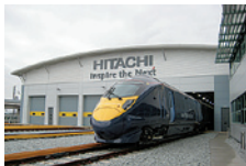
Ashford Train Maintenance Centre
