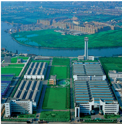
Hitachi Elevator (China) plant in Dashi Town, Guangzhou
