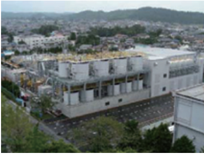
Advanced water treatment system (IPS Alpha Technology)
