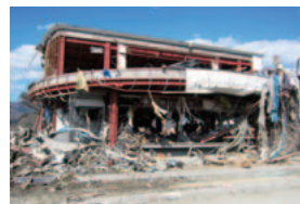
The tsunami devastated the Takata Branch, sweeping away the building front and ATMs.
