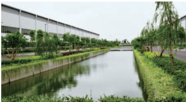
Pond where recycled water is stored after treatment
