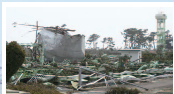
The tsunami wreaked pipes, wastewater intake equipment, pumping towers, machinery, and electrical equipment. Much equipment was destroyed.
