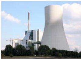
Ultra supercritical pressure coal-fired power plant*
